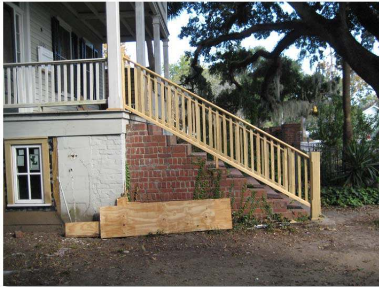
Front Stair Rails ready for priming
