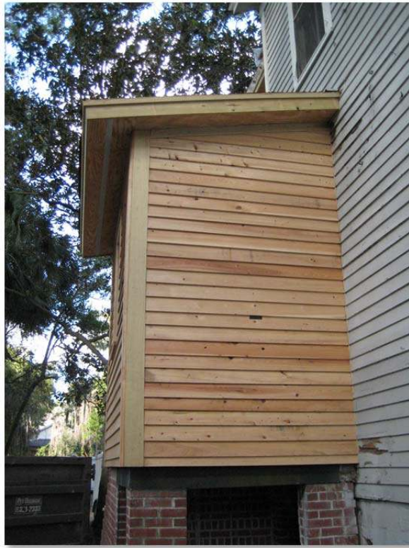
New Siding Matches up with Existing
