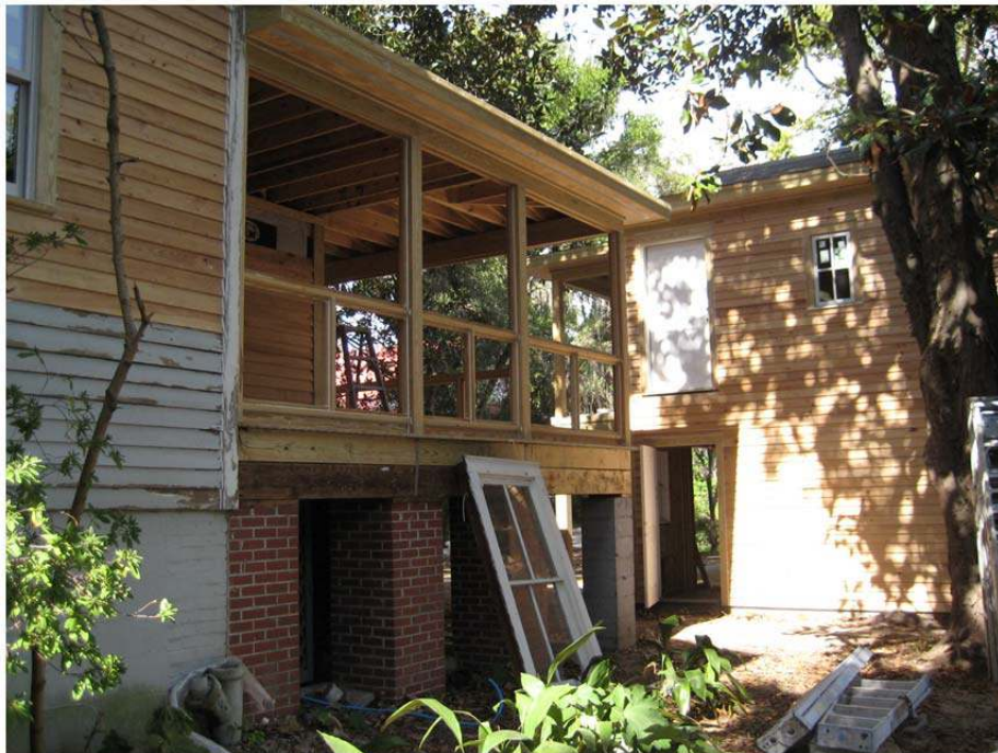
Screen Framing Installed waiting for the Bridge & pergola
