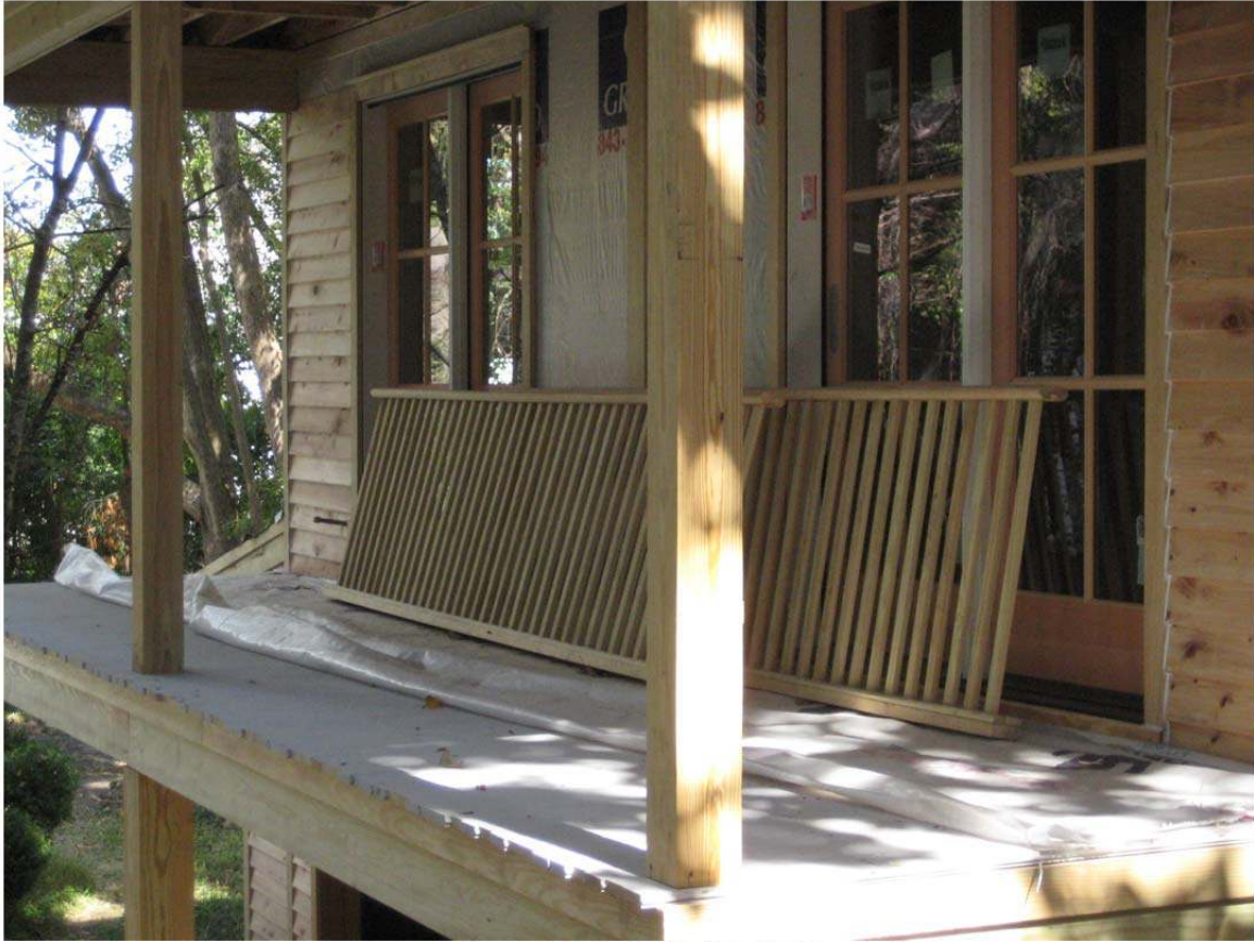
Apartment Porch Rail Prefabbed ready for priming
