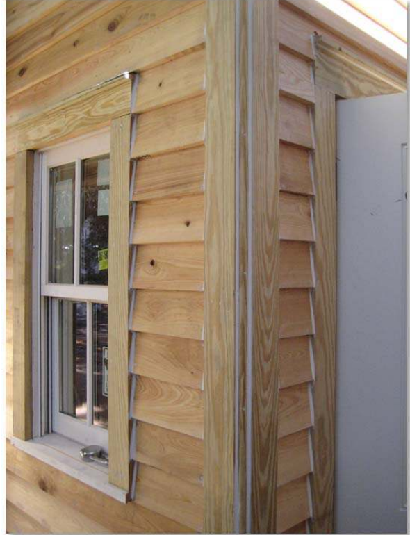
Siding & Trim Caulked tight nice neat work
