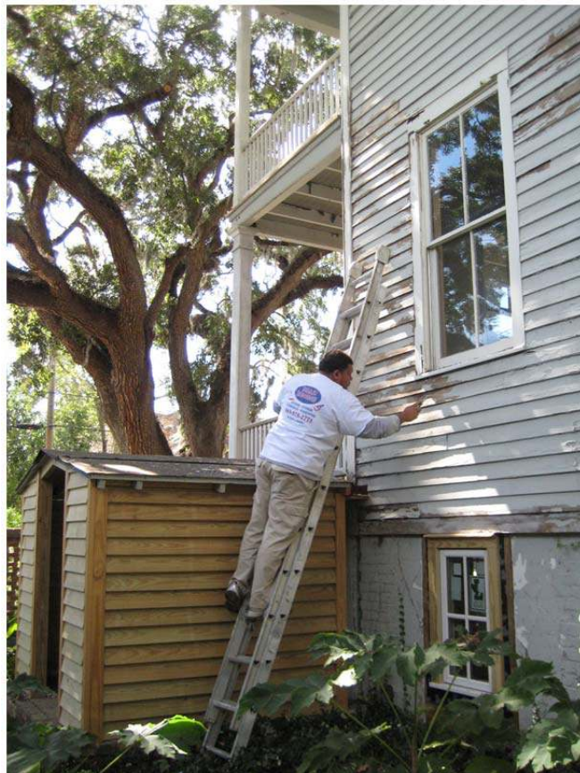
Orland Diaz (Diaz Painting) prepping existing Siding for Priming
