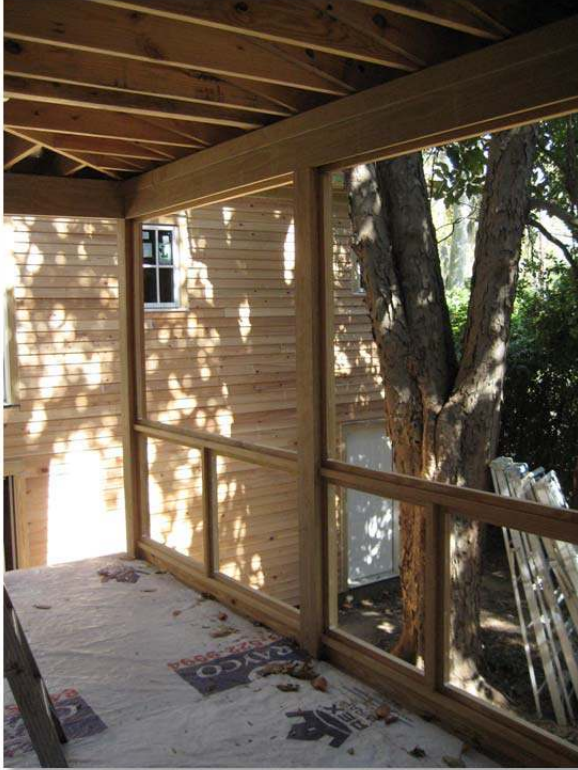
Screen Porch showing Screen framing
