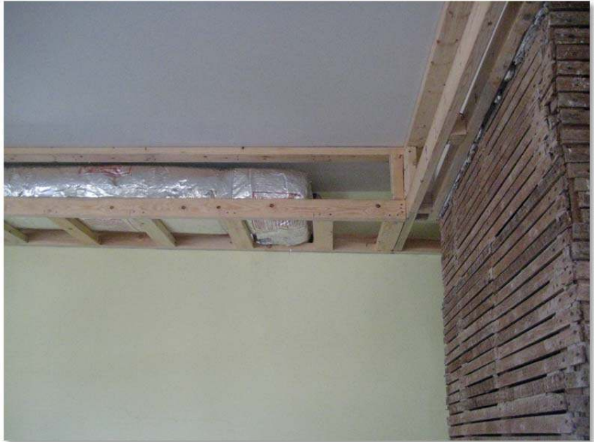
Neat transition out of Mechanical "Loft" to LR Soffit
